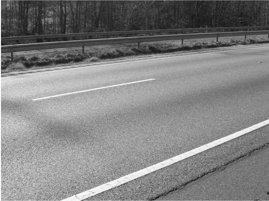
FIGURE 10 High-quality polymer-modified ultrathin wearing course, Burke County, North Carolina.
